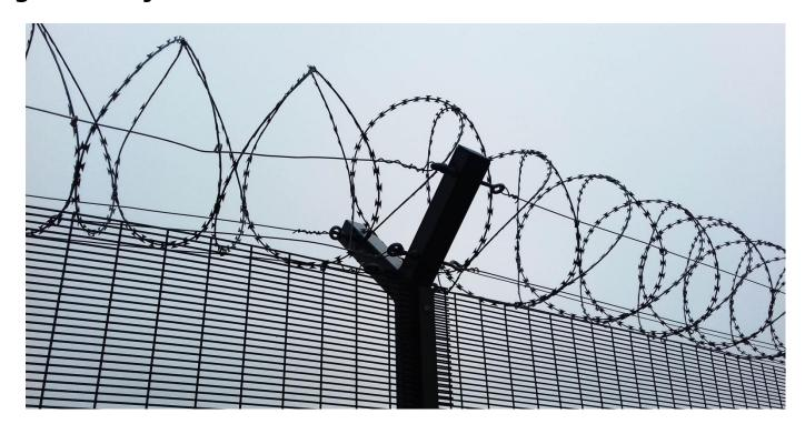
With the aesthetics of Sheerness Steelworks in mind the chosen contractor installed our black powder coated mesh and concertina razor wire around the perimeter of the site employing the highest levels of security. The installation required 4 sets of double leaf access gates and 1700 linear metres of 2.4m high Protek 358 prison mesh, aptly named due to its high security features.
